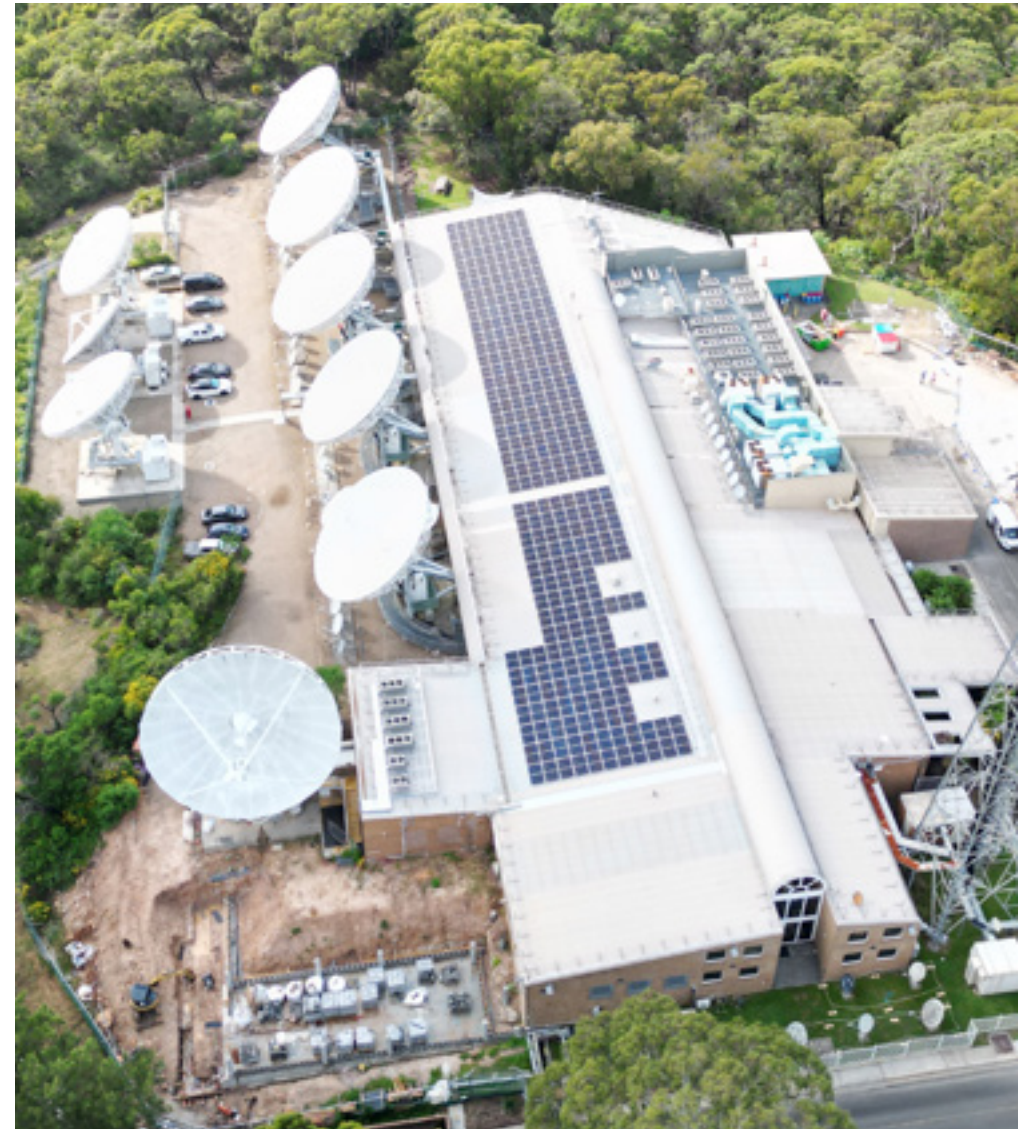
Solar panels at our Belrose satellite facility, NSW
