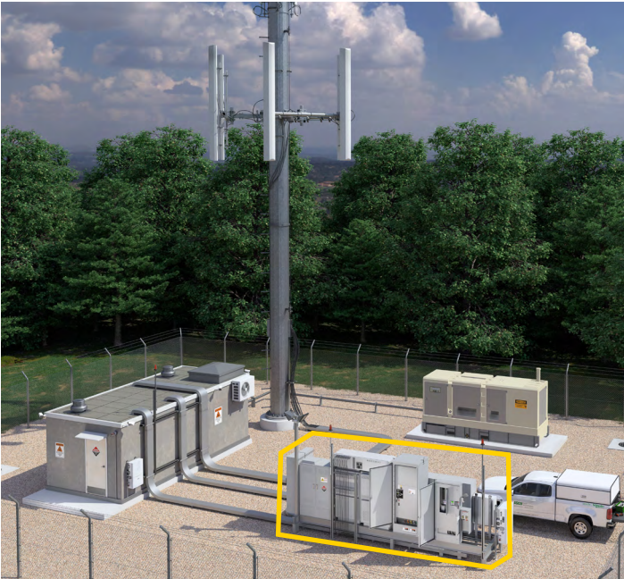
Automatic Transfer Switch
